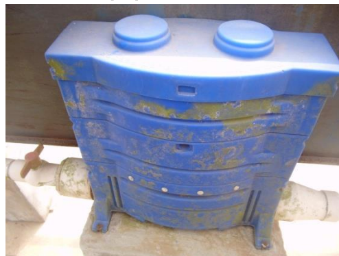
FIGURE 9: DISUSED CHLORINATION SYSTEM
