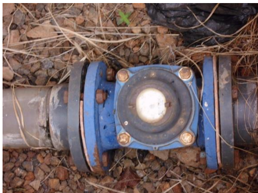
FIGURE 8: BROKEN BULK WATER METER
